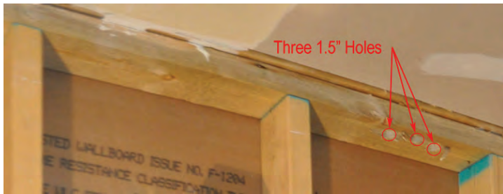
(c) Top Plate Configuration
