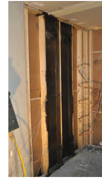
(b) Single Switch & Outlet Rear Overall
