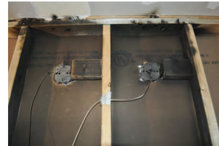
(e) Single Switch & Outlet Rear Top
