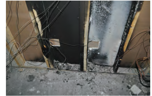
(b) Double Switch & Outlet Rear Bottom
