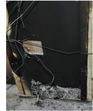
(b) Double Switch & Outlet Post Fire Rear
