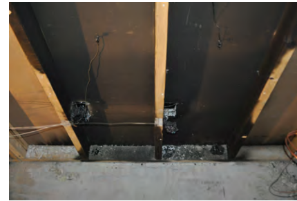
(c) Single Switch & Outlet Rear Bottom
