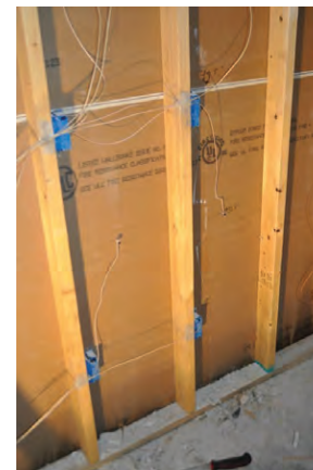
(a) Single Outlet and Switch Rear
