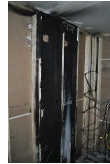
(a) Double Switch & Outlet Rear Overall
