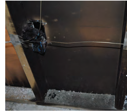
(a) Single Switch & Outlet Post Fire Rear
